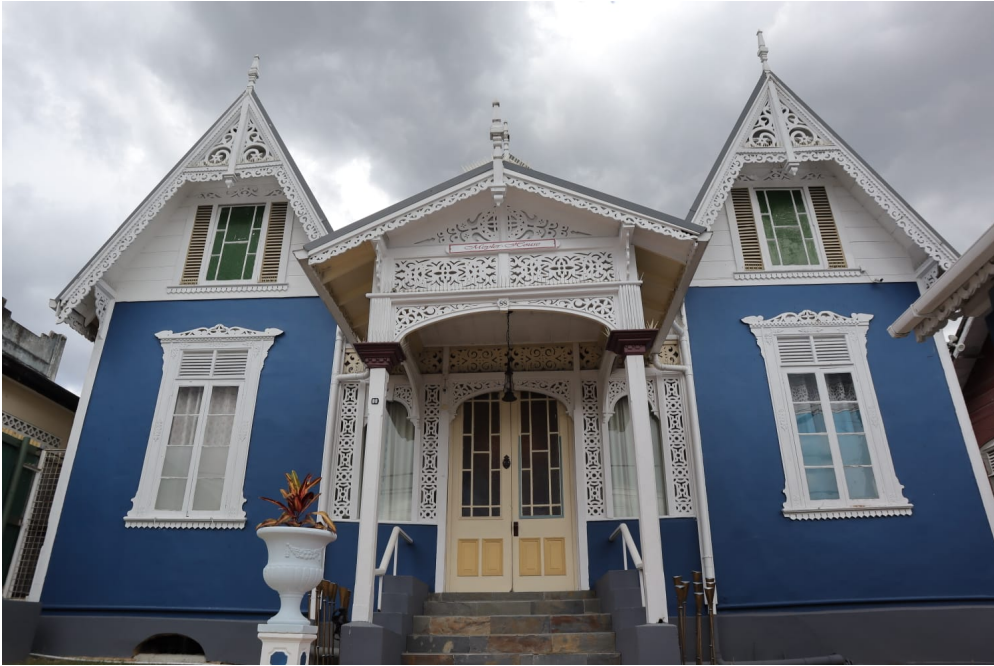
The pristinely renovated exterior of the Angelo Bissessarsingh Heritage House.
